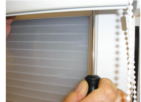
To remove the blind, push the lip of the bracket at the back of the cassette upwards using the head of a screwdriver. This will free the back of the cassette. Carefully remove to avoid damage to the blind.
